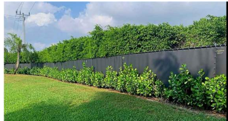
Chain link fence with protective shield
