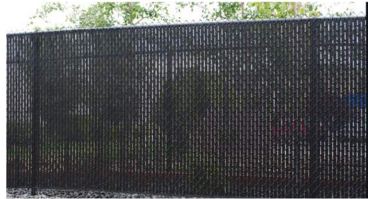
Chain link fence with slots
