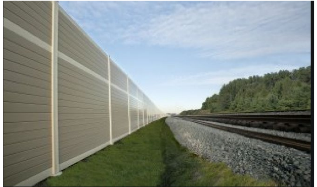
Pre-fabricated wall – Fiberglass panels
